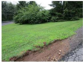
A bioretention system is proposed at the entrance of the property to reduce erosion and infiltrate the stormwater runoff from the parking area. A preliminary soil assessment suggests that the soils have suitable drainage characteristics for green infrastructure.
