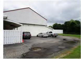
Porous pavement can be installed along the parking spots in the back lot of the building. The downspouts currently empty onto asphalt which is impervious and does not aid in infiltration. A preliminary soil assessment suggests that the soils have suitable drainage characteristics for green infrastructure.
