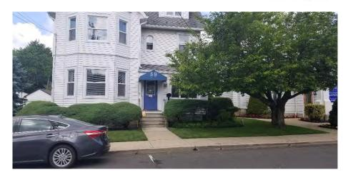
The downspouts along the north side of the building can be rerouted into downspout planter boxes to filter roof runoff. A small rain garden can be installed at the front of the building by redirecting downspouts into it. A preliminary soil assessment suggests that the soils have suitable drainage characteristics for green infrastructure.
