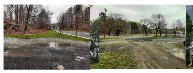
The southern corner of the parking lot can be converted to pervious pavement to allow for capture and infiltration of the stormwater runoff from the parking lot area. A bioretention system can be installed north of the parking lot to capture, treat, and infiltrate the stormwater runoff from the nearby grass and uphill area.
