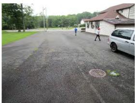
A bioretention system is proposed in the turfgrass to capture, treat, and infiltrate the west side of the parking lot and rooftop. Parking spaces on the east side of the parking lot can be converted to porous pavement to capture and infiltrate stormwater from the parking lot and rooftop. Planter boxes can be added to both entrances to capture runoff from the downspouts. A preliminary soil assessment suggests that the soils have suitable drainage characteristics for green infrastructure.
