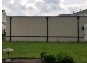
A bioretention system can be installed to infiltrate the water from three disconnected downspouts on the west side of the building. In addition, pervious pavement is proposed along the southeast corner of the parking lot to the parking lot's drainage area. A preliminary soil assessment suggests that the soils have suitable drainage characteristics for green infrastructure.
