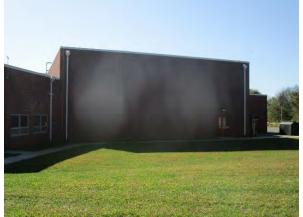
Bioretention systems can be installed in the north, west, and east corners of the building to capture, treat, and infiltrate rooftop runoff. Downspout planter boxes can be constructed along the south of the building to allow roof runoff to be reused. A preliminary soil assessment suggests that more soil testing would be required before determining the soil's suitability for green infrastructure.
