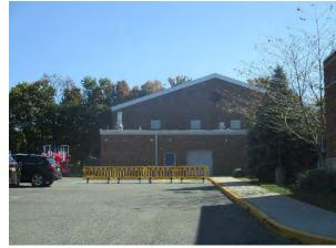
Porous pavement can be installed on the northern and eastern parking strips to capture stormwater from the parking lot. Downspout planter boxes can be constructed along the northeastern edge of the building to allow roof runoff to be reused. A preliminary soil assessment suggests that more soil testing would be required before determining the soil's suitability for green infrastructure.
