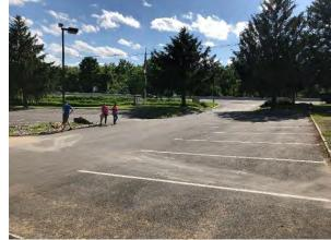
Pervious pavement can be installed in the southern parking lot to help remediate the pooling that occurs due to the pitch of the pavement. Bioretention systems can be installed west of the parking lot to allow for the capture of the parking lot runoff. A preliminary soil assessment suggests that the soils have suitable drainage characteristics for green infrastructure.
