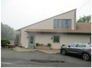
Connected downspouts can be rerouted into the existing planter boxes to be converted into downspout planter boxes. Downspout planter boxes can be constructed along the building to allow roof runoff to be reused. Porous pavement can be installed in the main parking spaces to capture and infiltrate stormwater runoff from the parking lot. A preliminary soil assessment suggests that more soil testing would be required before determining the soil's suitability for green infrastructure.
