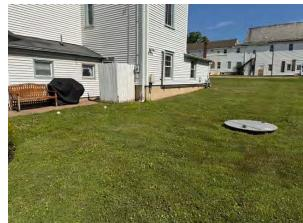
Three rain gardens requiring downspout disconnection and redirection can be installed in the grass areas around the building to capture, treat, and infiltrate stormwater runoff from the roof. A preliminary soil assessment suggests that the soils have suitable drainage characteristics for green infrastructure.
