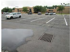
Two mowed detention basins at the east entrance can be retrofitted with rain gardens to capture, treat, and infiltrate stormwater runoff from the driveway and enhance pollinator habitat. Two sections of parking spaces can be converted to porous pavement to capture and infiltrate runoff from the parking lot. A preliminary soil assessment suggests that more soil testing would be required before determining the soil's suitability for green infrastructure.
